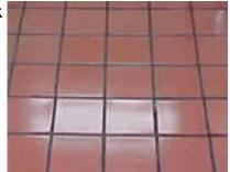
Quarry tiles are an unglazed ceramic material. They are particularly well suited for exterior paving due to their low absorption and resistance to freezing. This type of floor is one of the most durable on the market today. Esquire Services offers cleaning or stripping along with sealing or a wax finish. For best results, have your quarry tile & pavers brick sealed and use a neutral stone cleaner like StoneTech Professional<sup>TM</sup> Stone and Tile Cleaner available through Esquire Services.
